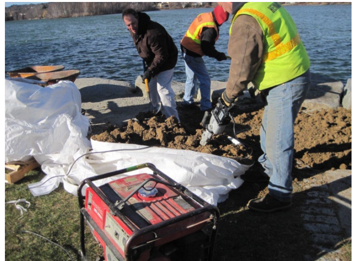
Using a jackhammer to break up clumps in one of the one-ton bags of StaLok® before installation
