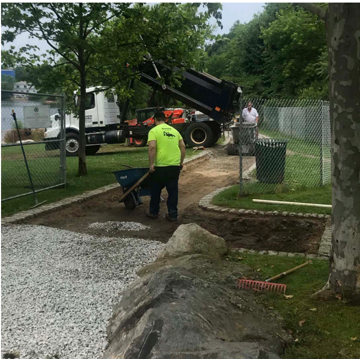
Haven Construction installed the porous path throughout the park, first with gravel, then crumbled tires
